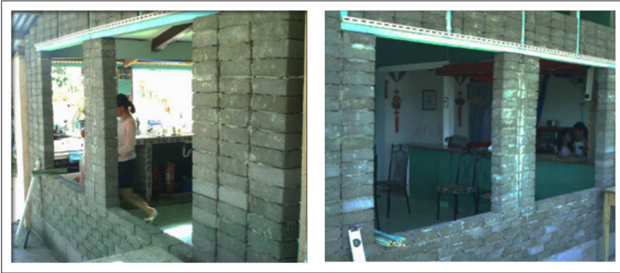
Figure 4. Frogged bricks showcased in building industry as external walls
